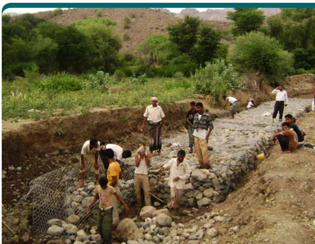
Building gabions to prevent the soil from erosion - Gol Madram - Al-Masaimir (Lahej)
