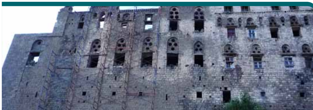
Restoration of Dar Al-Ezz Palace of 360 royal rooms – Jiblah (Ibb)
