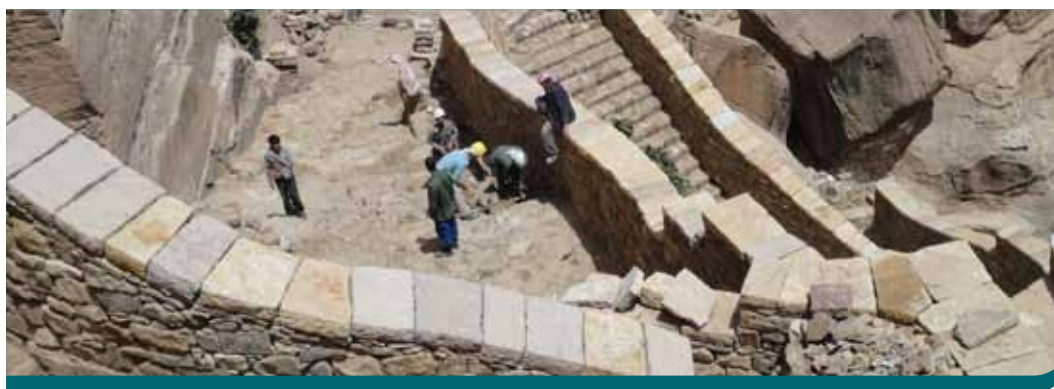
Restoration of the Historical Thula Fort Gate Project, providing employment opportunities (Amran)
